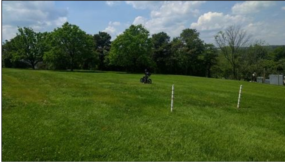
Figure 3. Site after soil backfilling and grass seeding.
