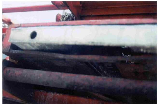
Figure 3: End view of ramp channel showing corrosion and damage
