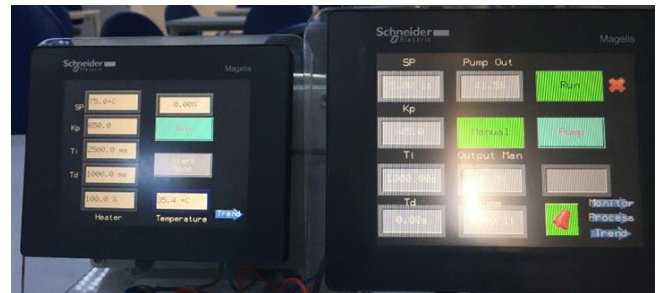
Fig. 5 PI and PID control parameters entry via HMI touch screen in automatic mode of control
