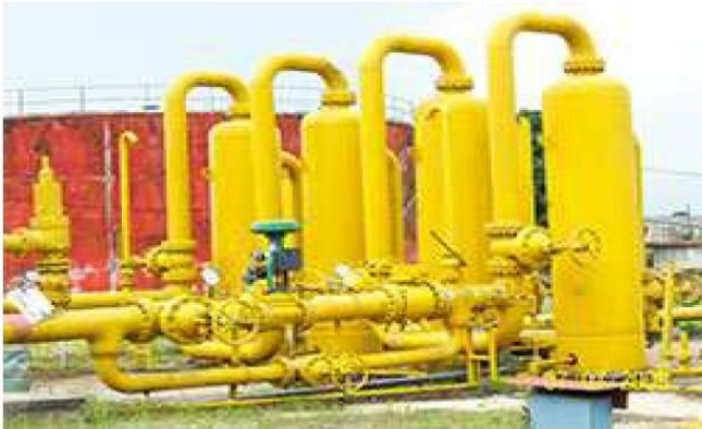
Fig 2: Piping Arrangement in Transcorp Power, Ughelli
