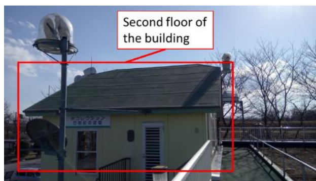
Fig. 3. Location of the second floor of the building, also showing the hand rails (lower)
