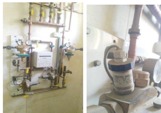
Figure.13 – Hospital O 2 Stations & sensors
