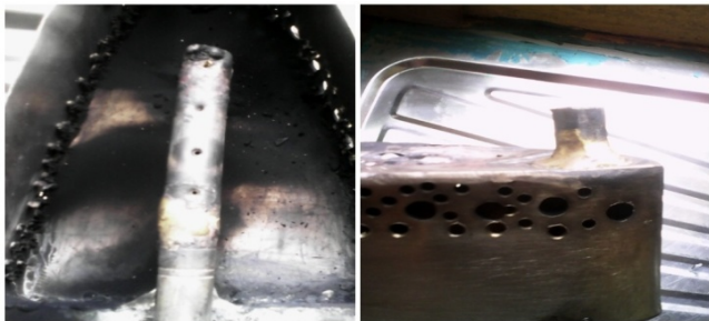
Fig 8. (L) Image of the burner. (R) Image of the chimney
