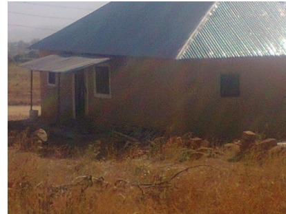
Plate 6: Building was Roofed in the Year 2013, still Shining in some Areas but getting Dull in Others.
