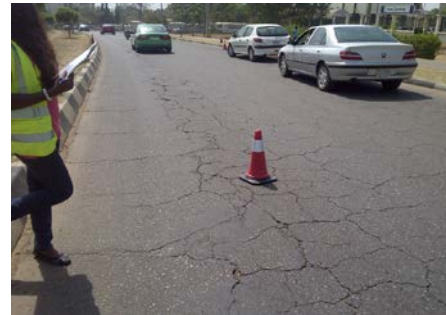
The existing road before rehabilitation
