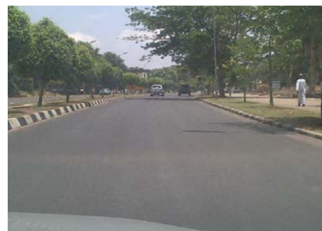
Newly rehabilitated road
