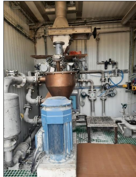
Figure 6. Hopper, the device where the polymer is mixed with water (Photo: author 2022)
