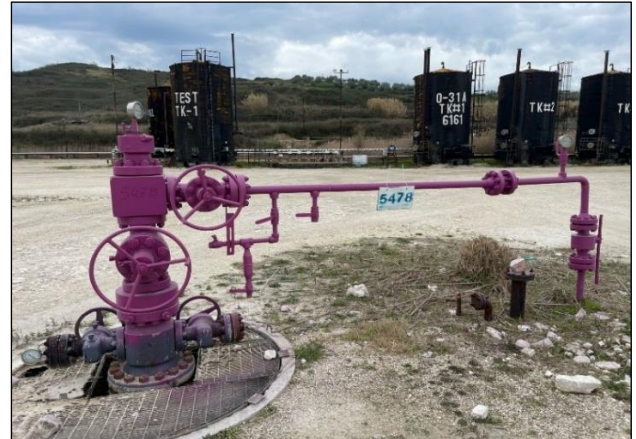
Figure 10. Injection well at the Patos-Marinéz oilfield (Photo: author 2024)
