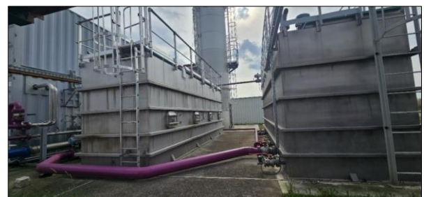
Figure 7. Deposit where the polymer solution is transferred, Patos-Marinza oilfield (Photo: author 2024)
