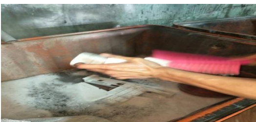
Fig.8 Checked completely entrance motor, power distribution board, sensor, etc.
