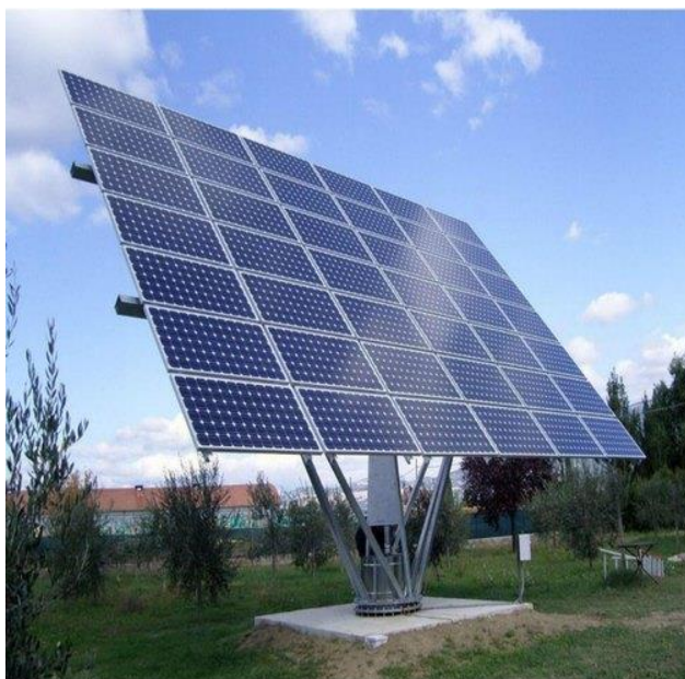
Figure 2: Single–Axes PV Tracker System aiming at the Brightest Point in the Sky
