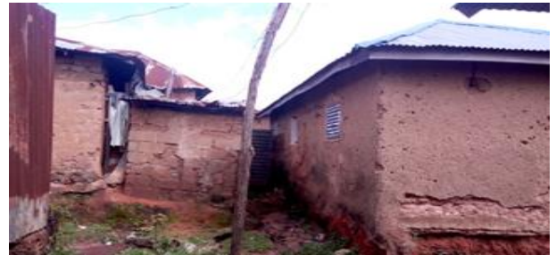
Fig. 4. Showing the housing condition in the area
