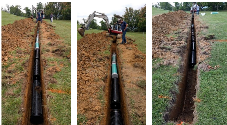
Fig. 2. 15.2 cm and 30.5 cm (6" and 12") diameter pipe samples being buried
