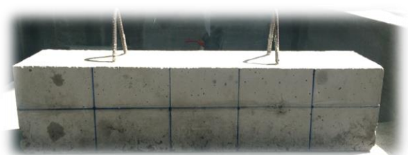
Fig.5 Grid marking on beam
