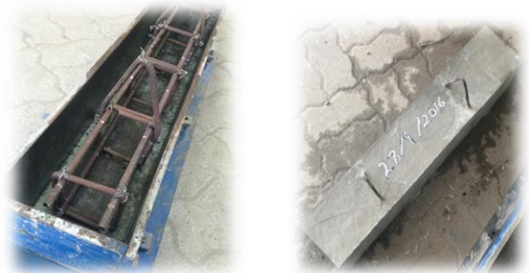
Fig.2 RC beam casting Fig.3 Finished beam
