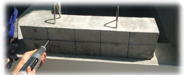
Fig.6 NDT for beam
