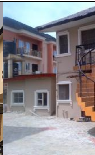
Figure 2 Oba Elegushi Royal Estate (Ileki-right), Ikate Elegushi, Lekki, Lagos Source: https://www.nigeriapropertycentre.com/for-rent/flats-apartments/self-contained/lagos/lekki/ikate-elegushi/showtype
