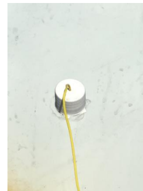
Plate 5. Glass cover thermocouples installation.
