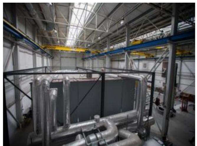
Fig. 7. View of duct-work of climate chamber under construction
