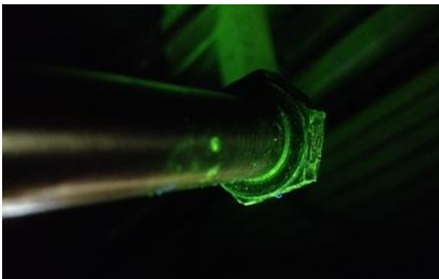
Fig. 12. Indication of cracks on a bolt
