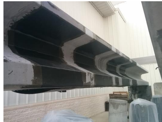
(a) Girder GF1.
