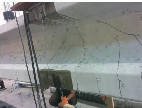
(b) Cracking at failure, GC.
