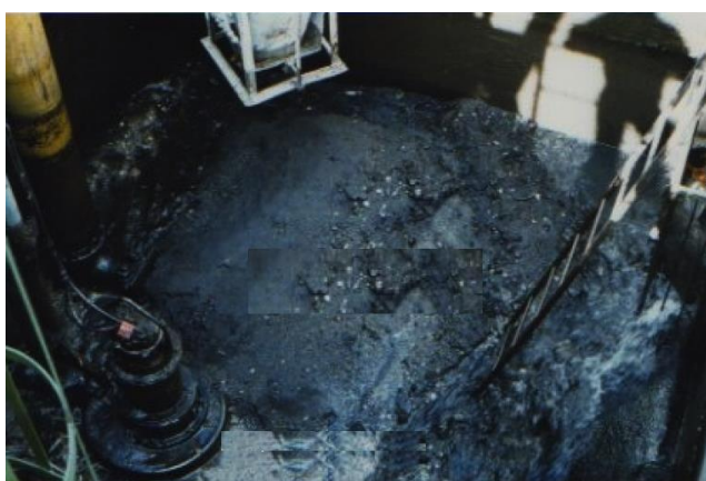
Fig. 6 - Solid material dragged into the equalization tank
