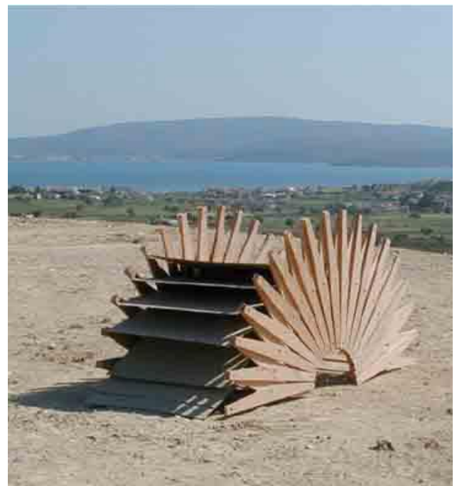
Figure 12: Retractable vault covered with rigid plates.
