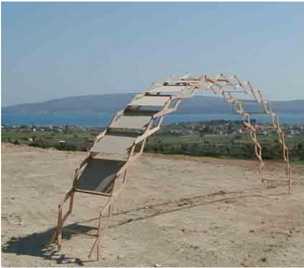
Figure 13: Retractable vault covered with rigid plates.
