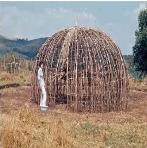
Fig 2. Structural Framework of a typical Fulani Hut in a Nomadic Fulani Settlement
