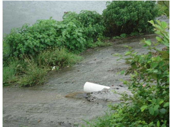
Fig.2: Storm sewer pipe out fall near Konapara
