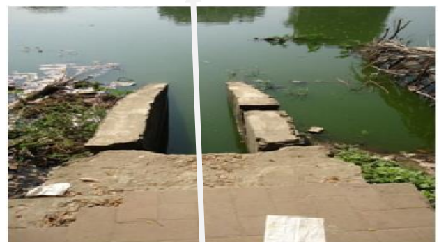
Fig 4: Open channel out fall at Lohar pool
