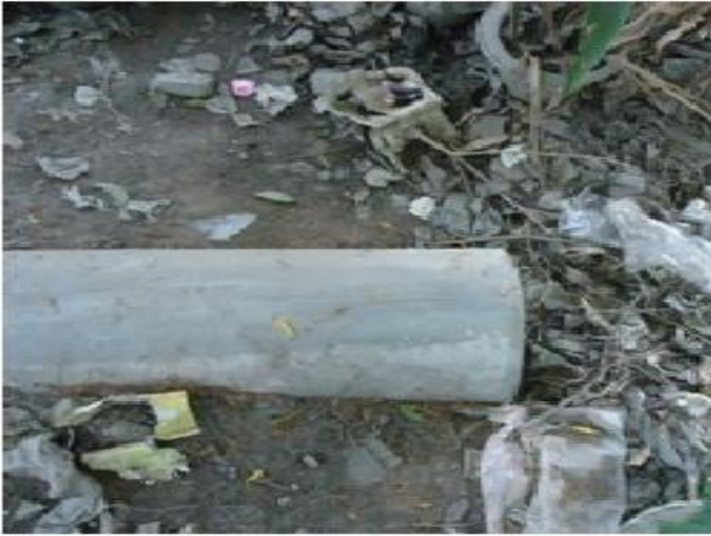
Fig 5: Sewer out fall near Staff Quarter
