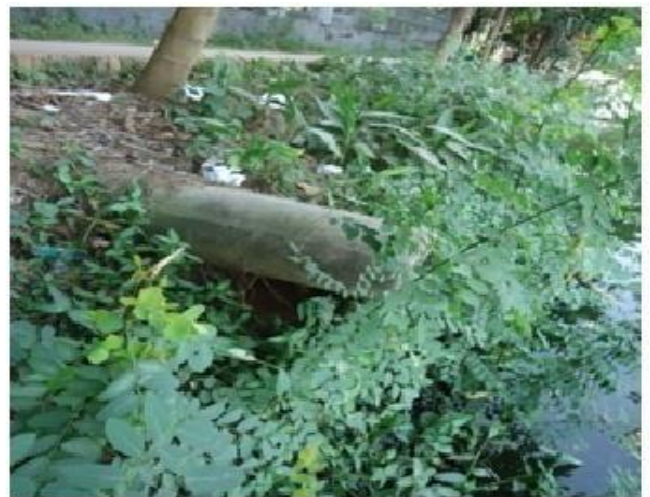
Fig 3: Storm Sewer out fall near Basher pool
