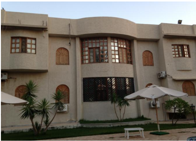
Figure 1: Northern façade of the building
