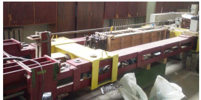
Fig. 4. Column in the strengthening process
