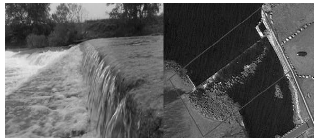
Fig. 5. A general view of a first site of the drainage channel 66 for a possible AST future development
