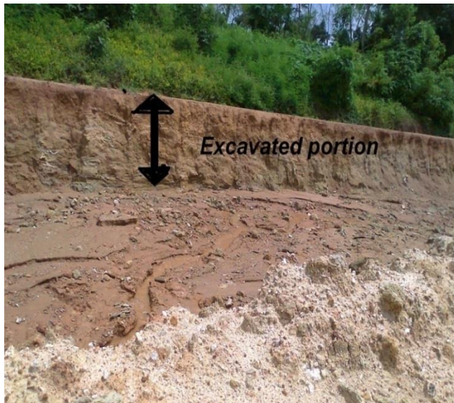
Figure 23: Excavated portion along the investigated road
