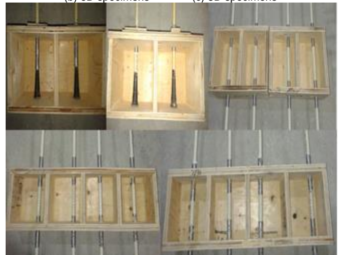
(d) Placement of GFRP bars in the forms Fig. 3. Dimensions and placement of GFRP bars in the forms (Dimensions in mm)
