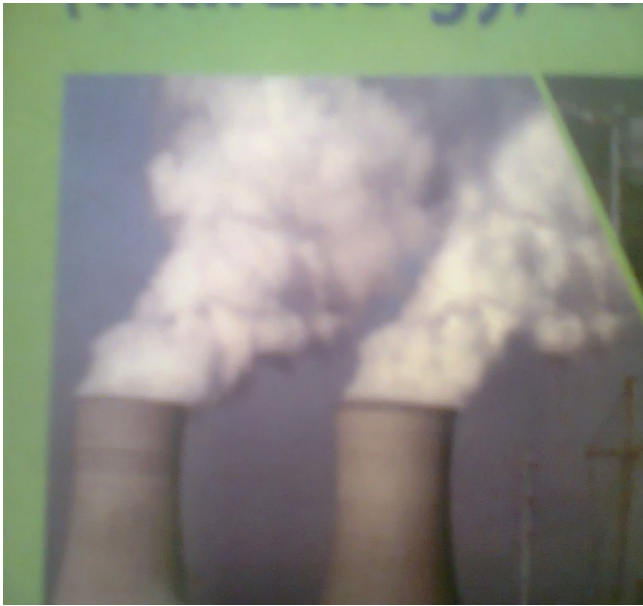
Fig.6: Huge Emissions from an Industrial Facility. Source: [8]
